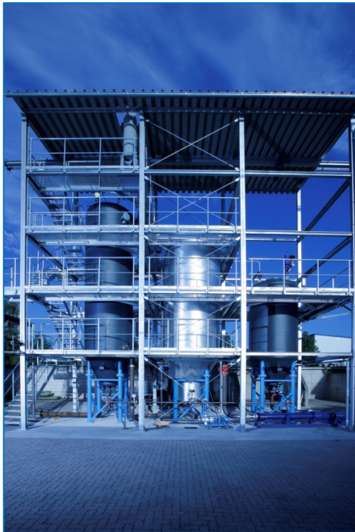
Figure 6: HTC demonstration plant for biocoal production at AVACO2.
